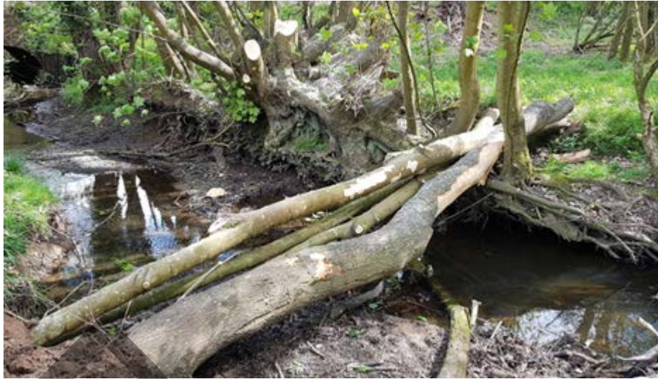
Figure 4: Leaky dam on River Bourne during installation in April 2019
