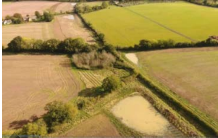
Figure 6: Field corner storage areas and riparian woodland planting as part of the Evenlode NFM project
